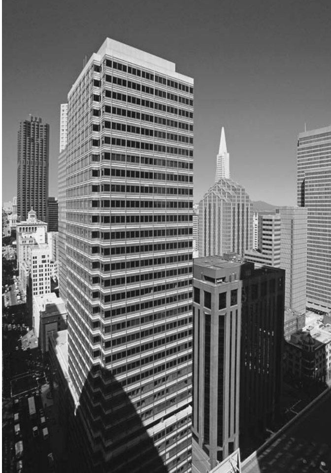
Figure 3.1 The 35-story office tower at 100 Pine Street in San Francisco is the first such building in California to receive LEED-EB certification, which should provide over time significant marketing benefits. Courtesy of Unico Properties.
